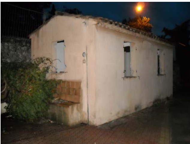
casetta in restauro
